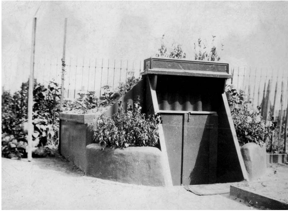
Figure 2.3. The modernistic Waker air-raid shelter in Dagenham. (London Borough of Barking & Dagenham Archives and Local Studies Centre)
